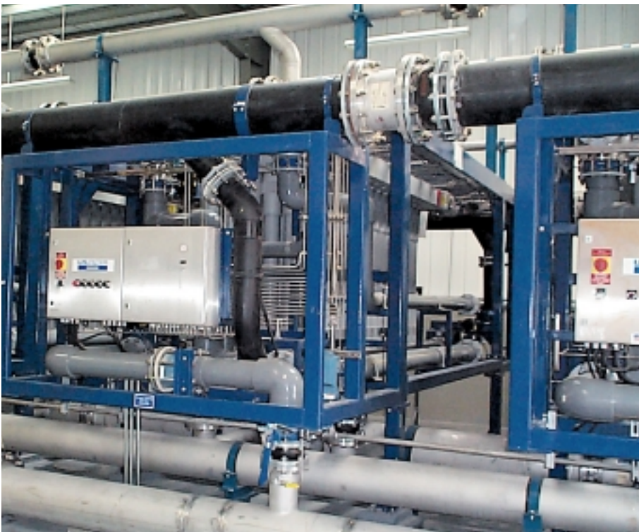
USFilter's Continuous MicroFiltration (CMF) system removes a wide range of contaminants from water.
