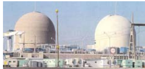
New Jersey's Salem Nuclear Power Station
