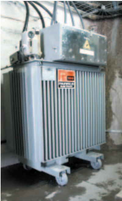
250 kVA Pauwels SLIM® with DuPont™ NOMEX® thermal technology.
