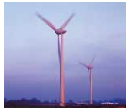
Pauwels SLIM® transformers are installed in Enercon E66/20_70 wind-turbines at Chépy, northern France. The transformers' reduced dimensions meant that they could be housed at the foot of the tower, thus saving the cost of separate buildings to house them.
