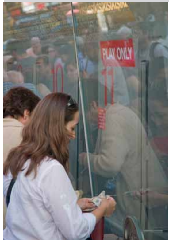
Structural glass made with DuPont™ SentryGlas® ionoplast interlayers is used for an internal load-bearing wall and front-facing ticket seller locations at TKTS in Times Square.
