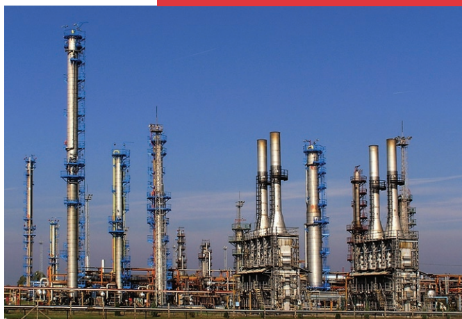
The MOL Algyő gas plant in Hungary
