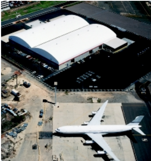
Quick construction and a durable cargo storage facility were the objectives met by Seaman Corporation's Shelter-Rite® fabric with Tedlar® for this United Airlines structure in Honolulu, Hawaii.
