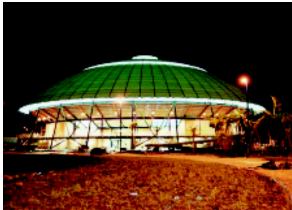
This multipurpose sports complex in Guanare, Venezuela will keep 7,000 fans comfortable for basketball. Its huge clear span tension membrane roof is Shelter-Rite® fabric with bright white Tedlar® PVF film.
