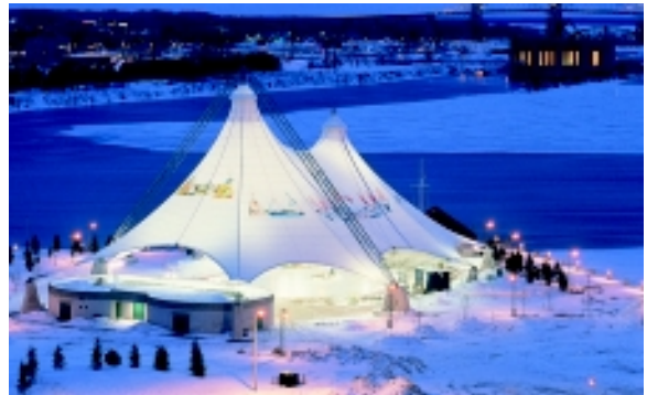
Shelter-Rite® fabric coated with Tedlar® provides protection from the elements in Sault Ste. Marie, Ontario, Canada. This pavilion houses hospitality and meeting space on an Indian reservation.
