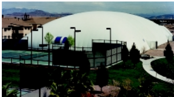
Construction costs were a major concern for the air-conditioned Green Valley Athletic Club in Henderson, Nevada, which accommodates four tennis courts under the air-supported structure protected by Tedlar®.
