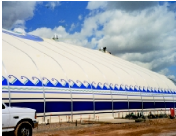
This 21,000 sq ft Indian Gaming Pavilion with attractive accent pattern provides a comfortable environment for thousands of visitors. The stressed membrane structure uses opaque Concord Cream Tedlar® to resist the constant blazing sun of central Arizona.
