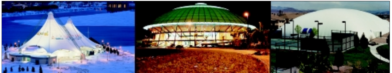
Figure 5. Three of the Many Fabric Structures Worldwide That Have Been Constructed to Meet Specific Usage Needs and Environmental Conditions
