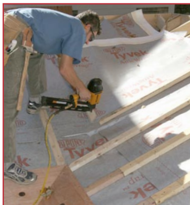
Nail furring strips over valley jack rafters
