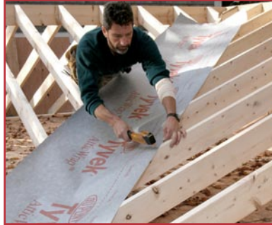
Line valley with half width sheet of Tyvek® AtticWrap™
