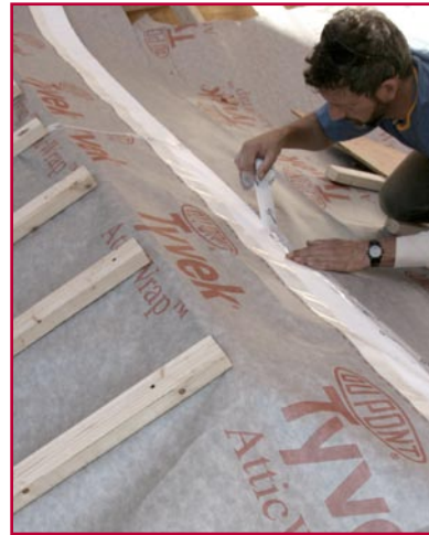
Fold Tyvek® AtticWrap™ over the ridge and over the membrane on the other side, then tape overlap
