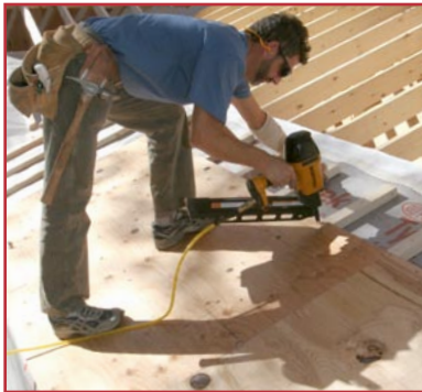
Nail roof sheathing over furring strips
