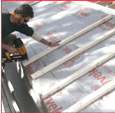
Nail furring strips over rafters
