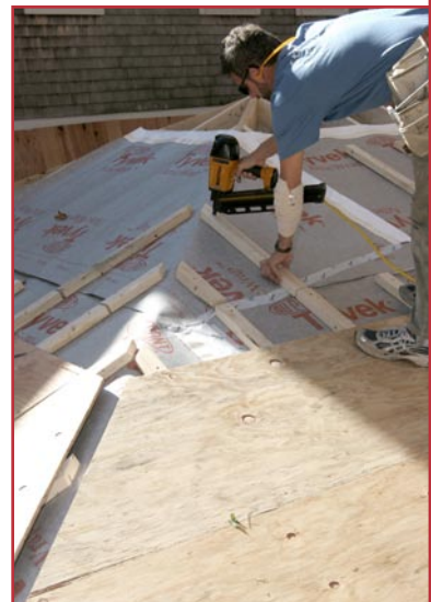
Fasten furring strips over hip jacks
