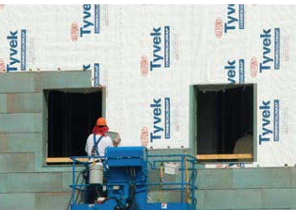
Acid-etched copper panels are installed over DuPont™ Tyvek® CommercialWrap® on the 10-story research facility building.
