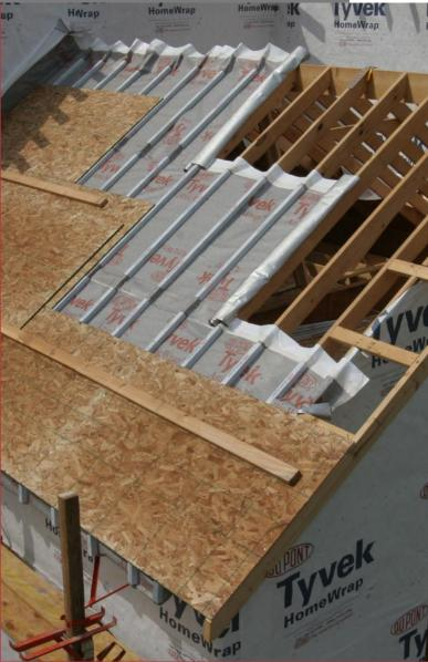
Tyvek® AtticWrap™ is rolled out in overlapping layers as work progresses from bottom to top (photo above) and can easily accommodate valleys and hips (photo left). The overlaps include an integrated adhesive strip (photo below) that allows for a tight airseal between successive layers, maintaining the integrity of Tyvek® AtticWrap™ as an air barrier.
